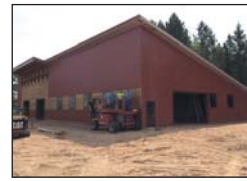
American Birkebeiner Trailhead and start line construction completed July 2016
